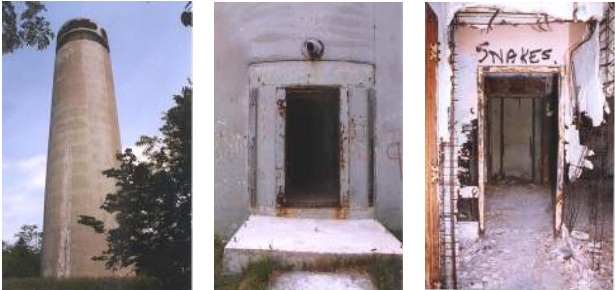
Cannonball's tower, door and entrance
