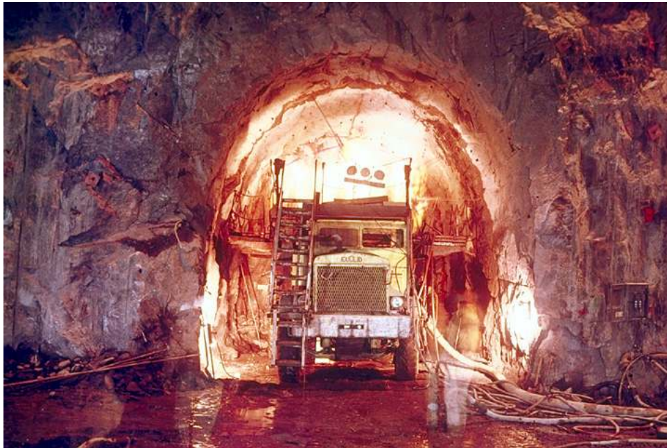
Cheyenne Mountain construction
