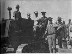
Butler on Marine tractor with a Chinese general and province governor, at Peichang, China, cooperating to build the Tientsin-Peking motor road in October, 1928
