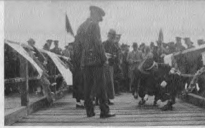
Driving the last four spikes into "Butler Bridge," built by the Marines at Peichang, in October, 1928, to replace a bridge on the Tientsin-Peking road washed out by storms
